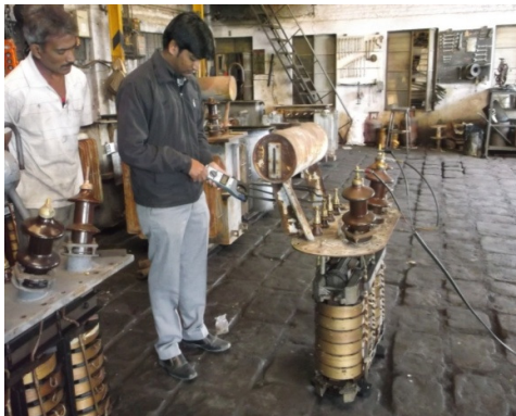
Fig.3. R,Y,B phase test of 63 KVA Transformer
