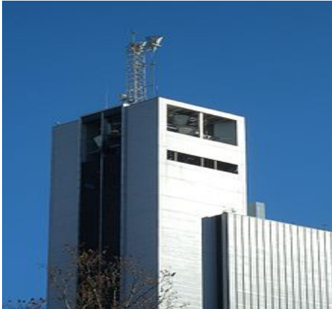
Telephone exchange with later antennas mounted higher for Antifade[1-5]
